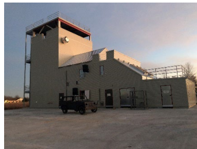
Bentonville Training Tower
