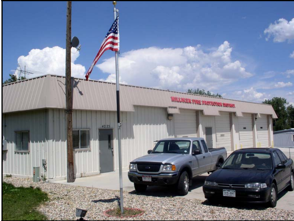
Figure 80: Milliken FPD Fire Station No. 2
