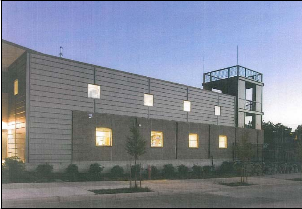
Figure 100: Headquarters Fire Station Side View
